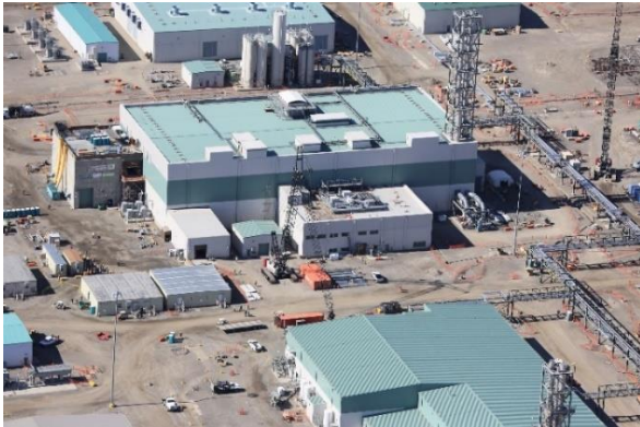
Aerial of the Low-Activity Waste (LAW) Facility. The LAW Facility will turn low-activity radioactive and chemical waste into glass to be permanently stored at Hanford.
