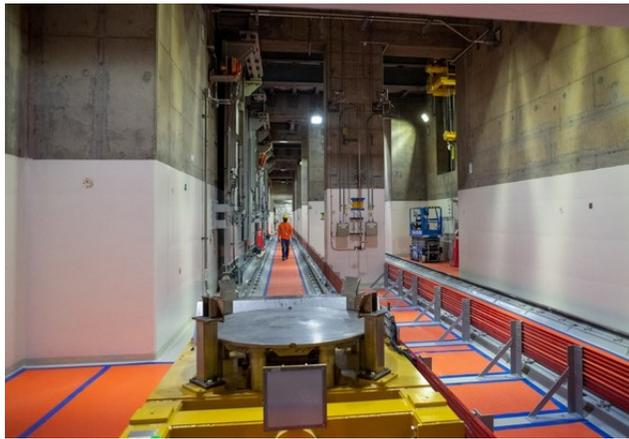
A Waste Treatment and Immobilization Plant worker walks along the transfer line in the basement of the Low-Activity Waste Facility. This system and all others in the facility have been completed and turned over for startup testing before being handed over to plant management for commissioning.
