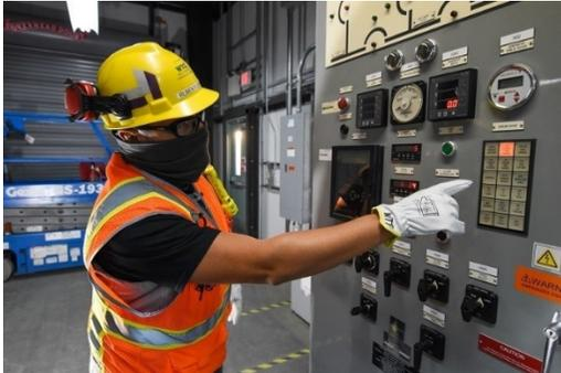
*Commissioning Technician Ruben Fuentes participates in the loss-of-offsite-power test for Hanford's Waste Treatment and Immobilization Plant from the switchgear building.*
