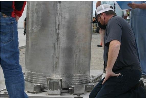
*Washington River Protection Solutions engineer Blake Chamberlain inspects the connection between an ion-exchange column and the bolts holding it in place on a concrete storage pad.*
