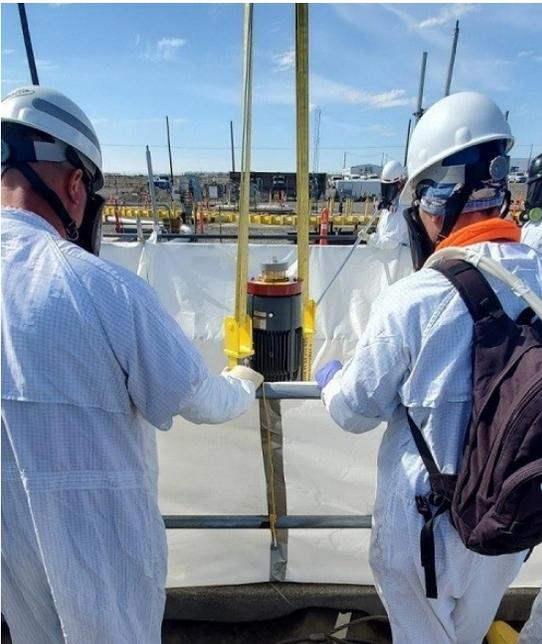
*Washington River Protection Solutions employees install a pair of pumps into tank AP-106, which will feed waste treated by a Tank-Side Cesium Removal system to the Waste Treatment and Immobilization Plant.*
