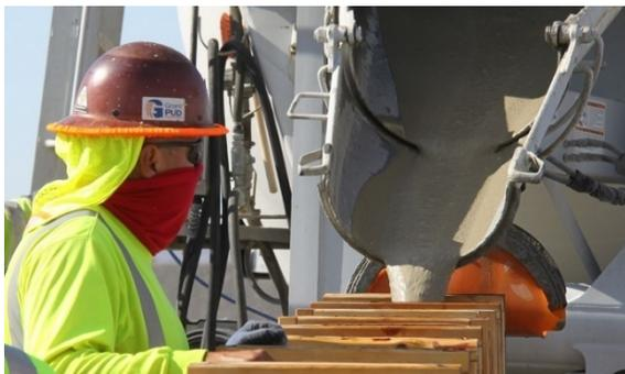
*Eddie Fernandez, field superintendent, monitors the flow of a test batch of engineered grout before it is used to stabilize aging underground structures in the 200 West Area of the Hanford Site.*
