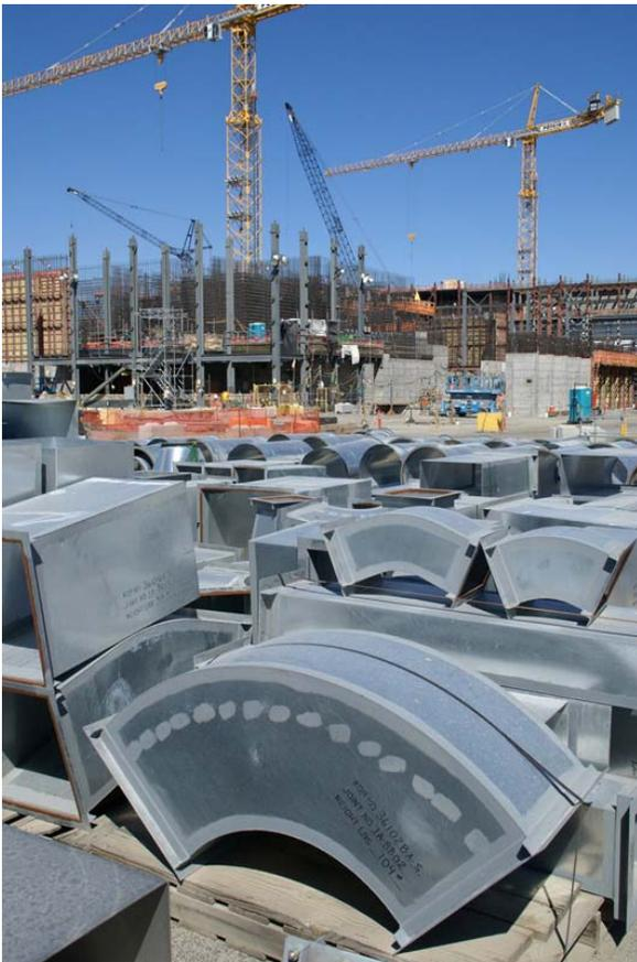
The High-Level Waste Vitrification Facility's HVAC design includes more than 600 tons of nuclear-grade materials, including some of the duct that is pictured above.
