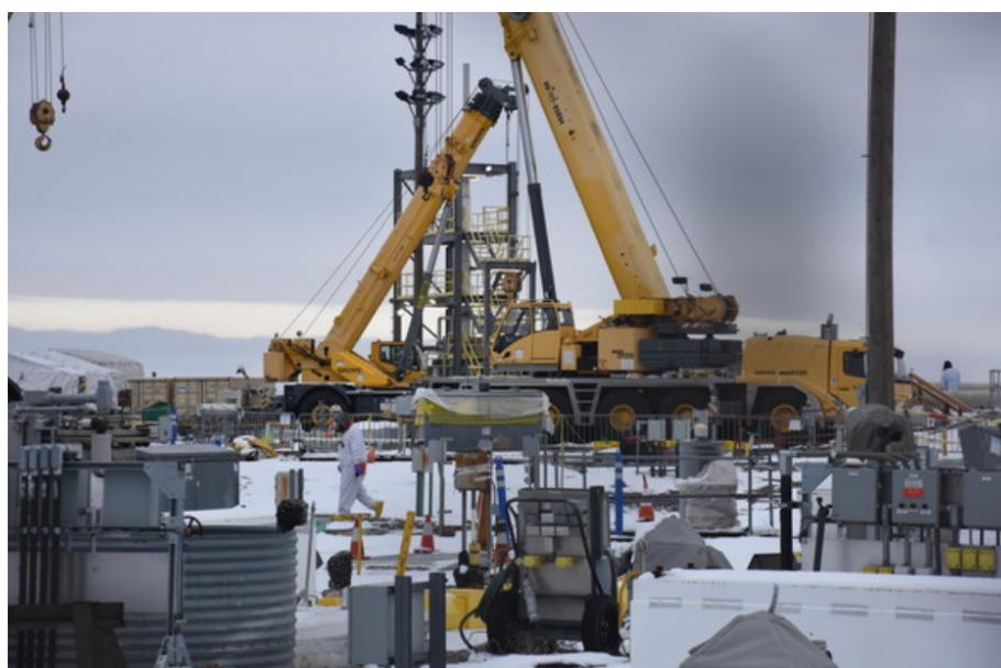
*Workers are retrieving waste from single-shell tank AX-104 at the Hanford Site. The waste is being transferred to a more robust double-shell tank for safe storage.*
