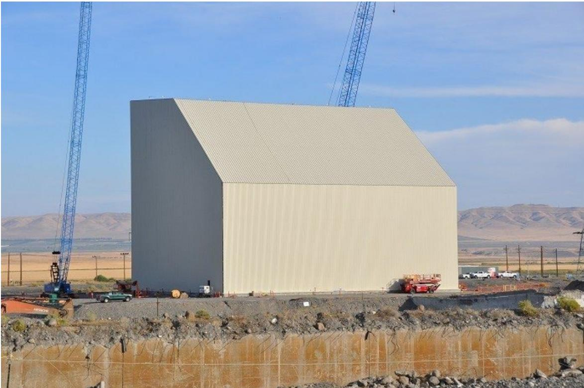
*Workers with Hanford Site contractor Central Plateau Cleanup Company recently completed construction of a protective enclosure, or cocoon, over the former K East Reactor building. The cocoon is designed to protect the reactor building while the radioactivity in the deactivated reactor core decays over the next several decades, making it safer to complete disposition of the reactor in the future.*
