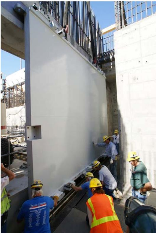
The High-Level Waste (HLW) Vitrification Facility shield doors are 8 inches thick, 15 feet tall and 18 feet wide. Two of the doors weigh 50 tons, and two weigh 14 tons. Setting these doors will allow construction to continue above and around them.
