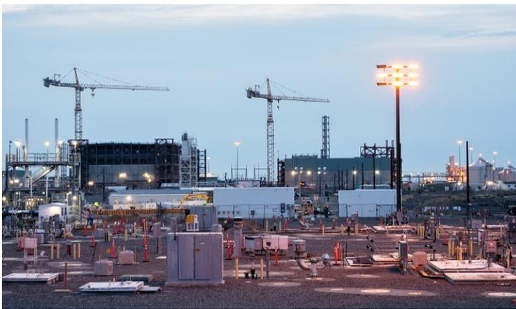
*The white enclosures of the Tank-Side Cesium Removal system are visible adjacent to the Hanford Site’s AP Tank Farm. In the background is the Waste Treatment and Immobilization Plant, where waste pre-treated by TSCR will be heated to 2,100 degrees Fahrenheit, mixed with glass-forming materials, and poured into stainless steel containers for disposal.*
