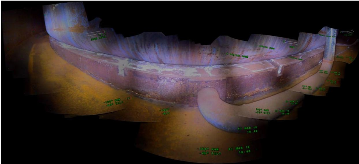
Figure 3. Double-Shell Tank Annulus Composite Image, Lower Tank and Annulus Floor
