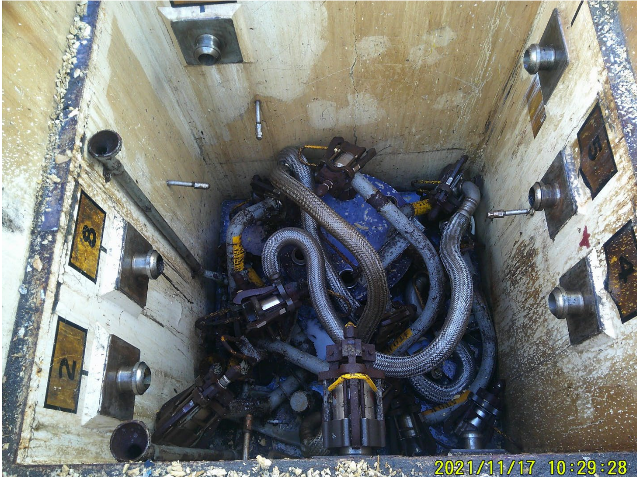
Figure 2. Image of a typical SST pit (with shield blocks removed)
